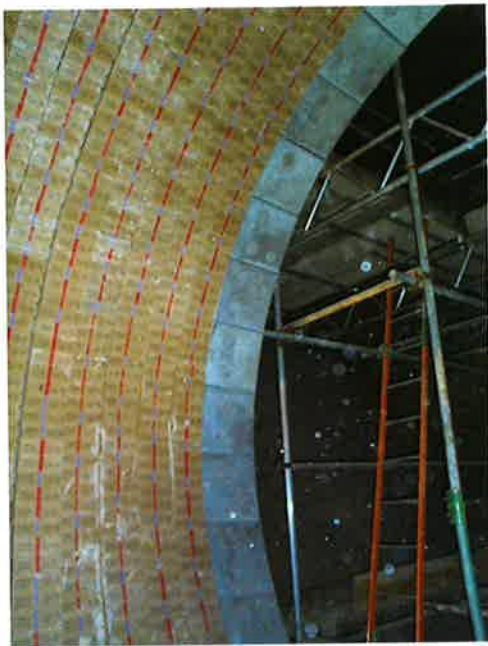
Fig. 3 Precast kiln outlet nosering system (Courtesy of Hanson UK)
