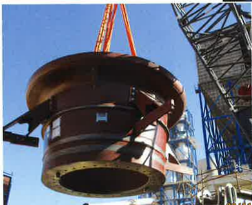
The lifting of the cement mill table (above) and the completed mill (right)
